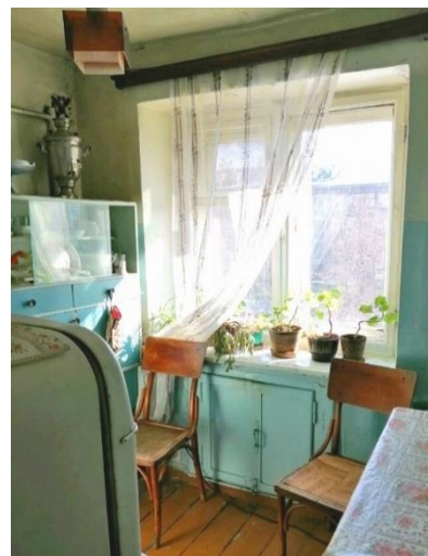
Figure 4.2A cold cabinet under a wide window sill in the presence of an electric refrigerator.
